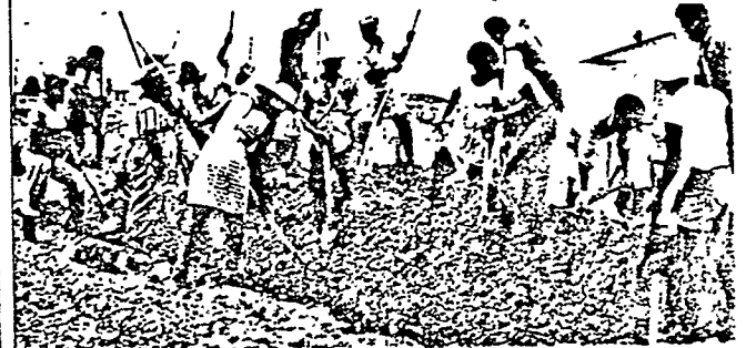
A group of Guyana Developers at work at the site of Guyana newest community Co-op at Elizabeth Hall. These developers are spreading materials on a roadway at the site.
